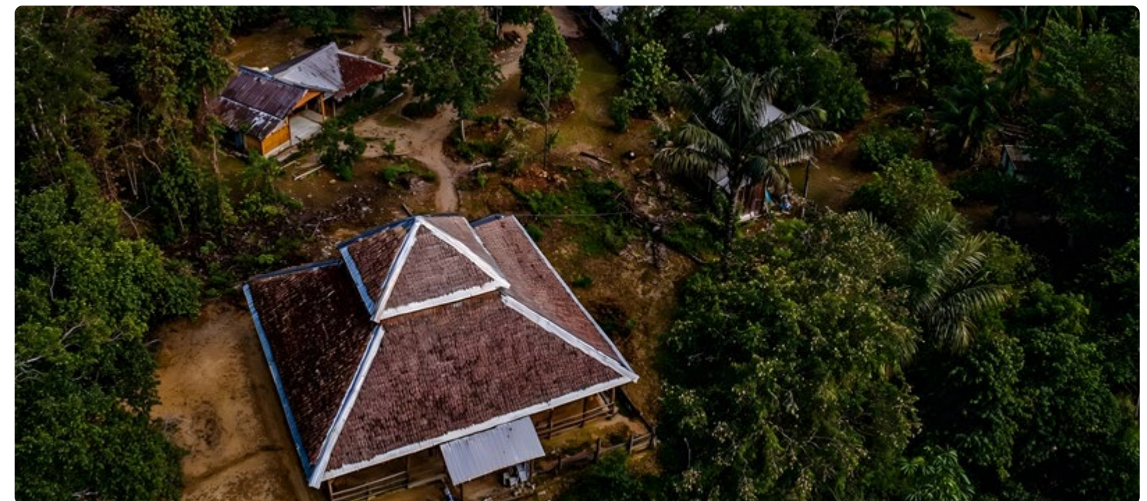
Aerial photograph of part of the Santa Casa structure. Photo: Pedro Adnet
