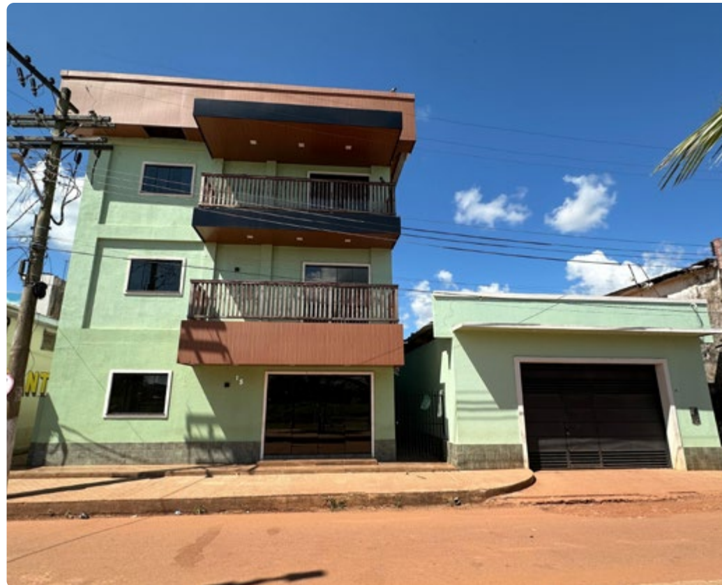
View of the facade of Hotel Floresta after the completion of the renovation. Photo: Pedro Adnet
